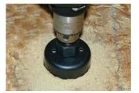
2. Drill hole in floor using hole saw.
