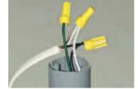
4. Connect receptacle wires to cable. Be sure to match wire colour(s).
