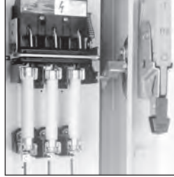
Type MCS Disconnect Switch with fixed-depth, flange-mounted handle
