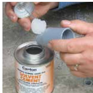
Apply a uniform coat of cement.
