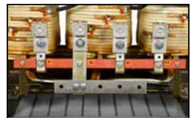
Expanded neutral bar for multiple customer connections
