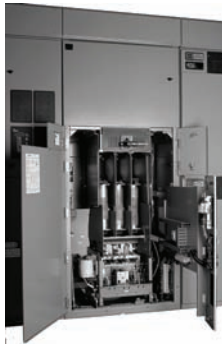
50L7 Vacuum Retrofit
