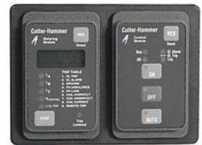
Advantage Device Panel with ACM and Metering Module
