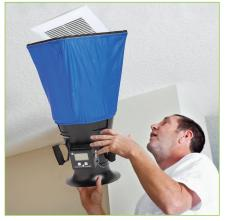
Balometer used to verify installed performance
