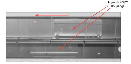
**Step 4.** Install the next fitting. Measure and cut DS4000 Base at the closest score short of the fitting. Install DS4000 Base and tighten Coupling screws.
