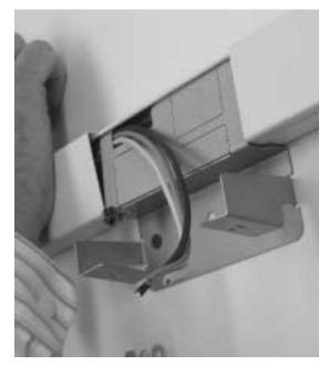
5. Wire device and mount on bracket.
