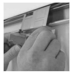
4. Feed wire through twistout and snap on raceway covers.
