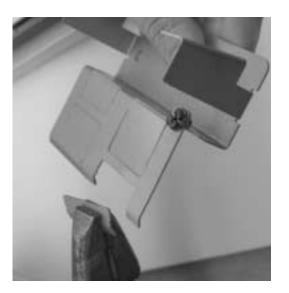
**3.** Attach bracket to the wall using #8 (5/16" [7.9mm] head size) flat head fastener or equivalent.
