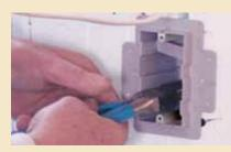
**STEP 2:** Insert the INEXO box into your opening and push the 'teeth' into place until you hear the 'click' – so you know your box is secure. If you are positioned next to a tie, you can utilize two of the 'teeth' on the non-tie side and use the flange holes on the opposite side to screw into the plastic tie.
