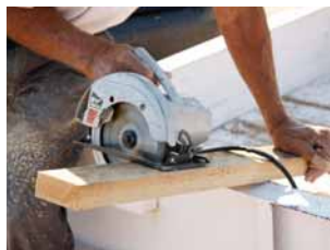
Construction Site Application
