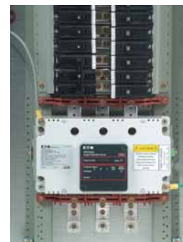
In this installation, the SPD Series is mounted directly to the panelboard's bus bars. This type of installation will provide the best possible surge protection by minimizing the connected lead length.
