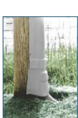
Carlon PV-Mold is a non-metallic pole riser system designed to protect communications or power cable installed on poles.
