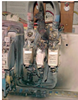
Fig. 5.8.1 – Unsuccessful disconnection of current resonance
