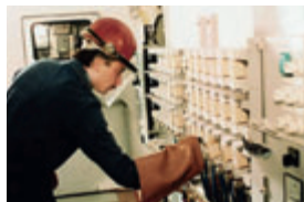
Fig. 3.2.4 – Actuating LV HRC fuse links under load
