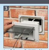
Install the supplied NM cable connector and wire. Insert the clean IN BOX into the sleeve.
