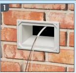
Mortar in adapter sleeve. Pull wire and tie off to loop in adapter sleeve.
