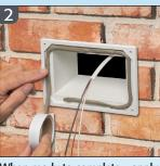
When ready to complete... apply supplied caulk as shown and press around edges of adapter sleeve.
