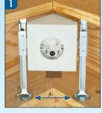
For proper fan/fixture installation, use supplied template to level and position brackets between rafters. Remove captive screws on sides of brackets and use to attach FBX900 assembly to rafters.
