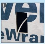
Cut a 3-1/4" x 5-1/2" hole in substrate. Pull wiring.
