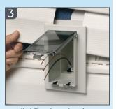
Install siding, inserting the cut ends of the siding under the outer flange of the IN BOX.
