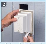
Apply the supplied caulk around back edges of flange, Install NM cable connector and wire, then press onto surface.
