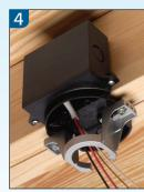
4. Pull wires through knockout. (Installation of drywall not shown.)
