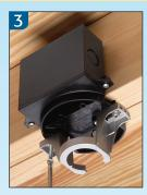
Remove captive bracket installation screws. Use them to mount fan/ fixture bracket.
