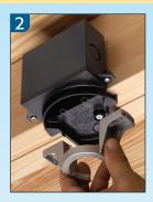
Position mounting bracket over locator posts to assure proper position.
