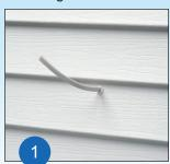
Select location for light fixture and caulk opening around cable.
