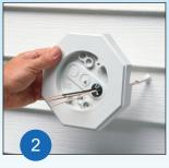
Remove knockout from electrical box and insert cable connector. Push cable through connector and position mounting block onto siding.
