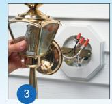
Secure mounting block with provided screws. Install fixture per manufacturer's instructions.
