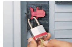
Multi Pole Breaker Lockout
