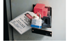
Oversize Breaker Lockout
